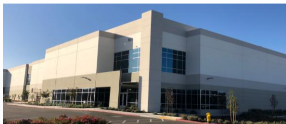
New Livermore Manufacturing Center
