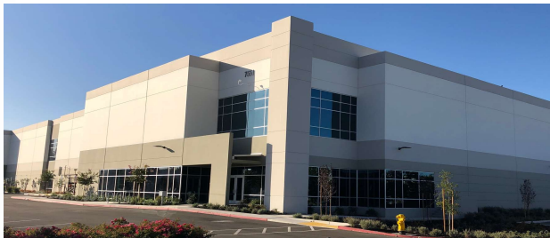
New Livermore Manufacturing Center
